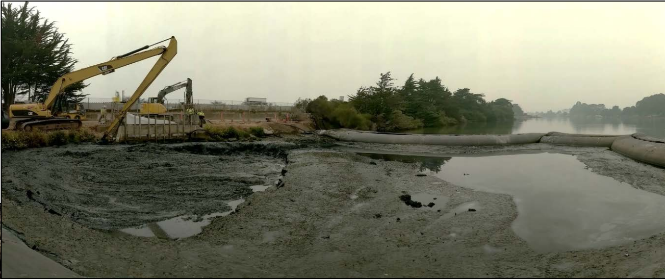
Lagoonside sediment removal and coffer dam
